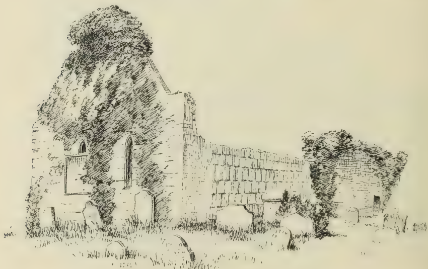
FIG. 1386.—Rosyth Church. View from North-East.
